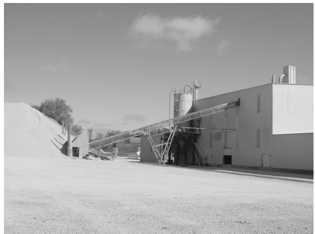
Weeping Water Plant
